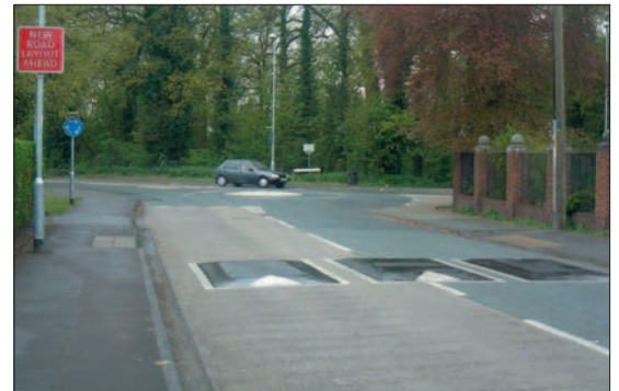
Photo 2.5.1: Mini-roundabout in traffic calmed area
