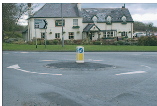
Photo 2.1.5: Street furniture on a domed central island in tarmac creating a small roundabout, not a mini-roundabout
