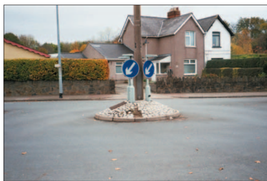
Photo 2.1.4: Street furniture on central island creating a small roundabout, not a mini-roundabout
