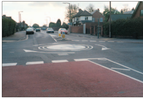
Photo 2.1.3: Non-conforming concentric rings
