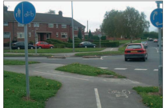
Photo 3.11.2: Mini-roundabout with off-highway cycle facilities
