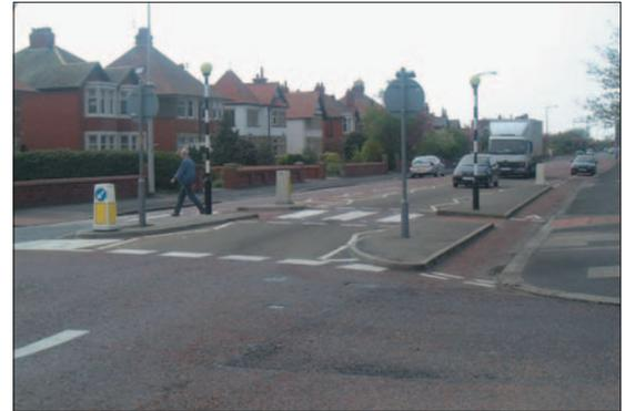
**Photo 3.7.3: Mini-roundabout incorporating segregated cycle facilities and zebra crossing**
