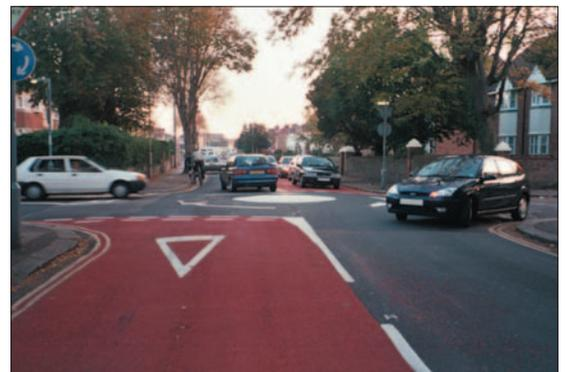
Photo 4.2.10: Mini-roundabout with red anti-skid
