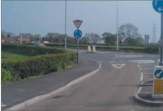
**Photo 3.6.1: Example of mini-roundabout within 40 mph speed limit with constrained approach**
