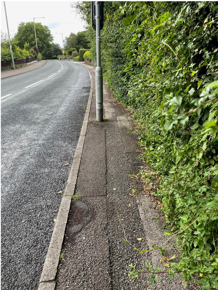
**Footpath heading north from Slater Lane junction towards the bus stop illustrated above - very narrow pavement obstructed by lamp-post.**
