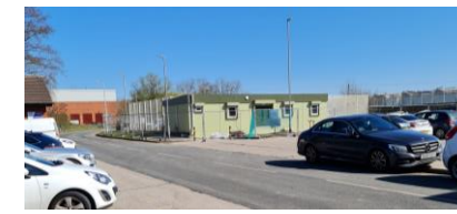
Existing portacabin office and car park
