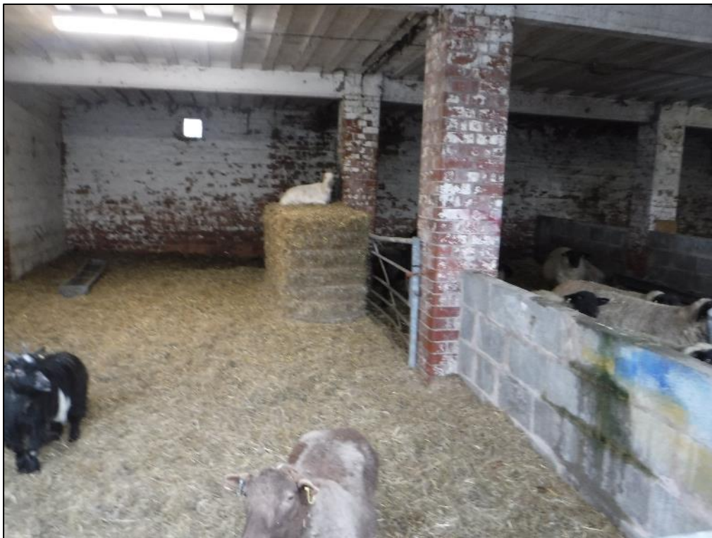
Photo 6 – Internal room of Building B5.
