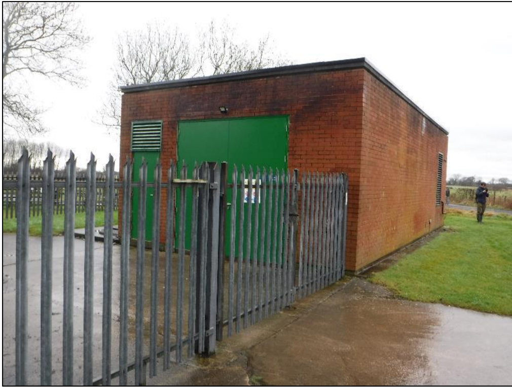
Photo 9 – South aspect of Building B8.
