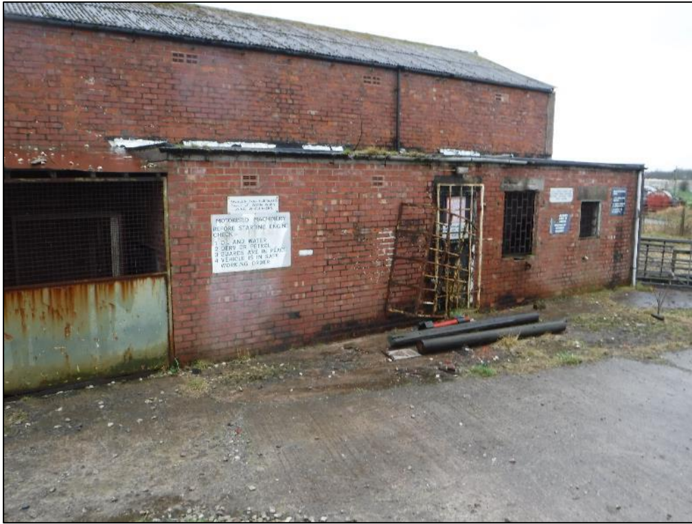
Photo 13 – North aspect of Building B10.
