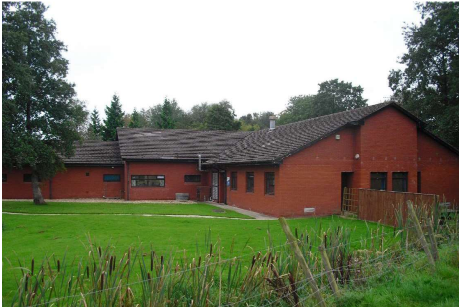
Photo 16. Building for which records of a common pipistrelle maternity roost were returned from LERN, recorded in 2009/ 2010 (TN36)
