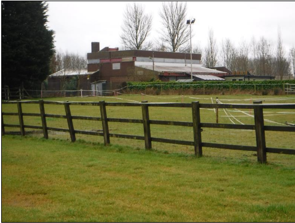
Photo 7 – North-west aspect of Building B6.
