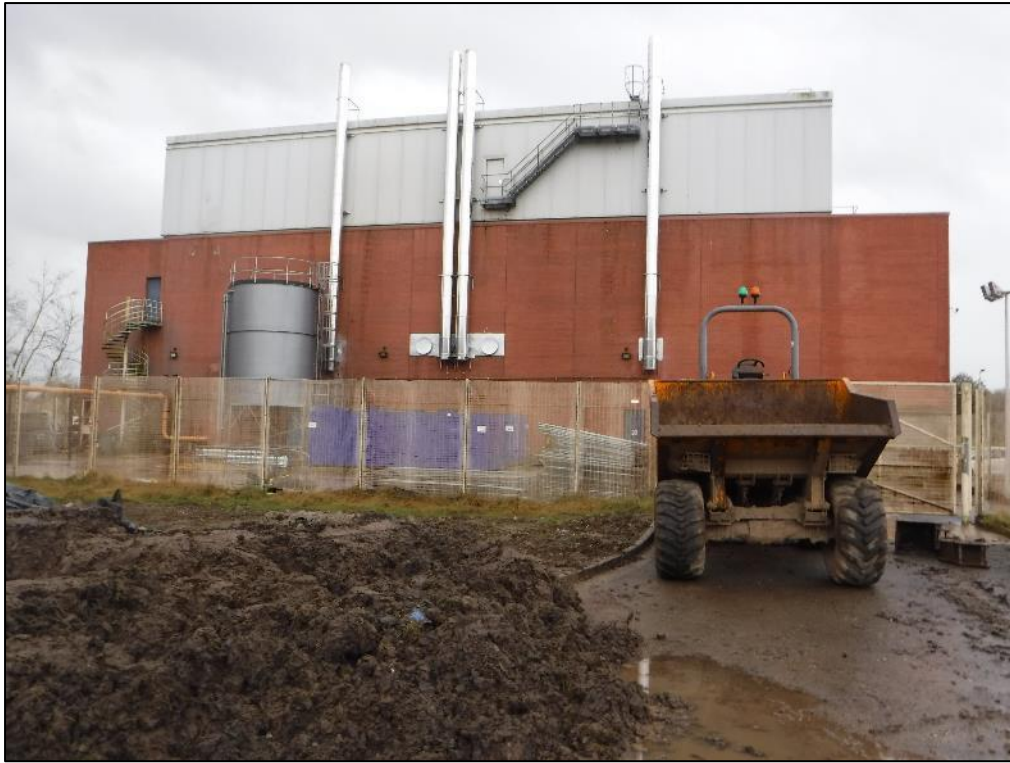
Photo 11 – North aspect of Building B9.
