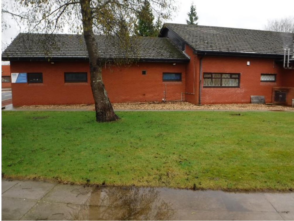
Photo 17 – North aspect of Building B15.
