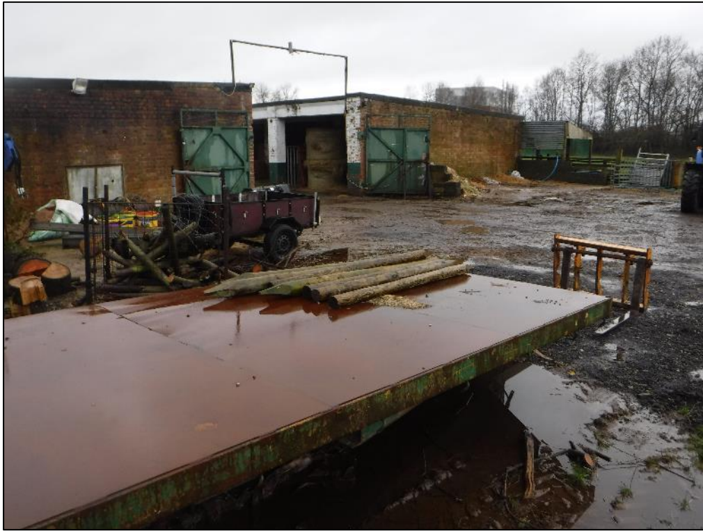
Photo 5 – North aspect of building B5.
