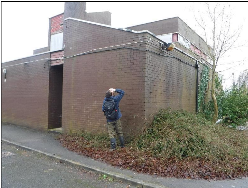
Photo 8 – South-west corner of Building B6.
