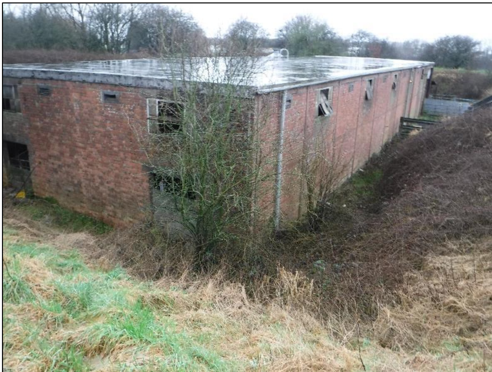
Photo 14 – North-east corner of Building B11.
