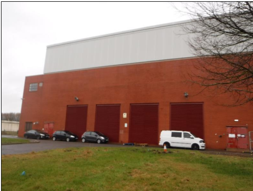
Photo 10 – South aspect of Building B9.
