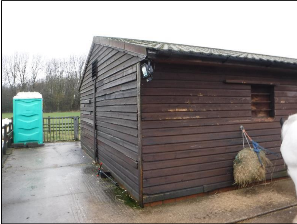
Photo 1 – South gable of Building B1.
