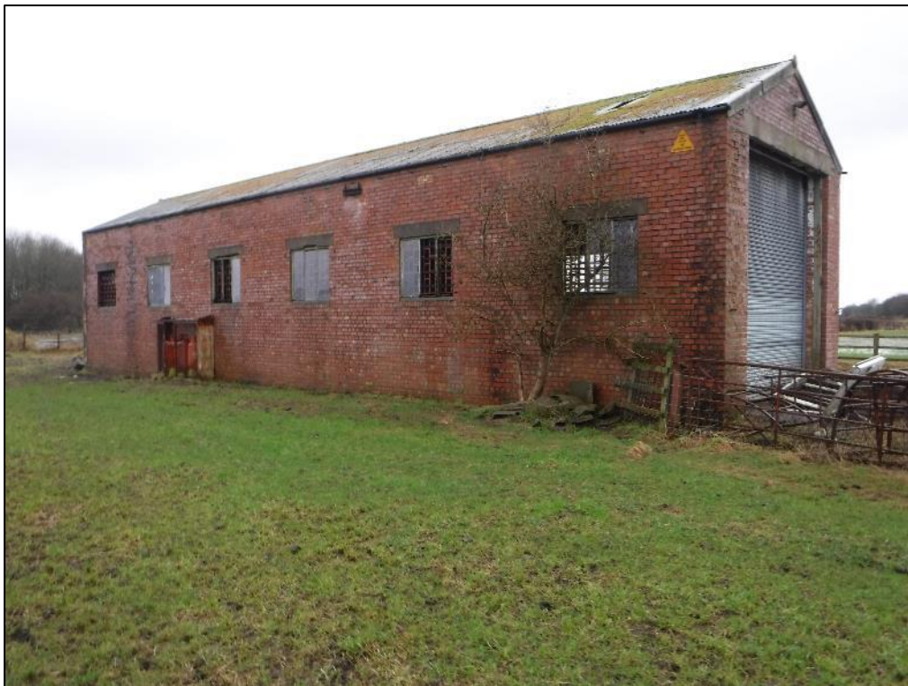
Photo 12 – South aspect of Building B10.
