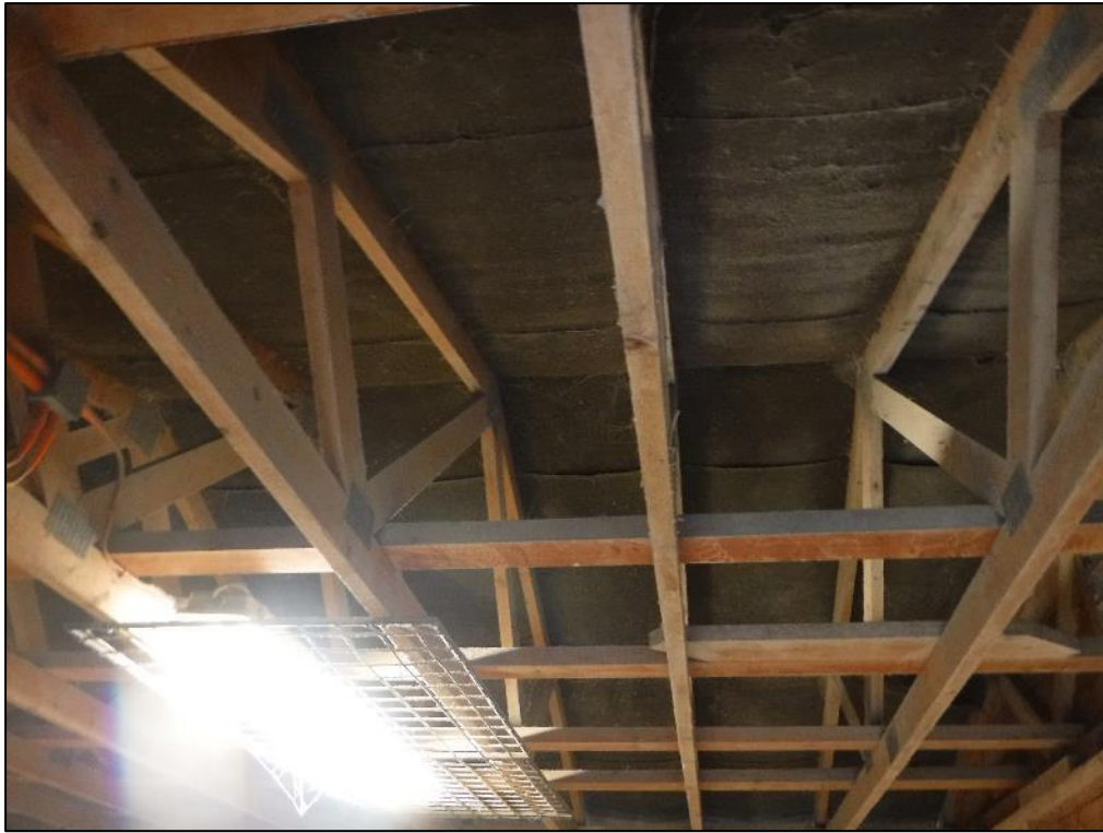
Photo 3 – Underside of roof of Building B1.
