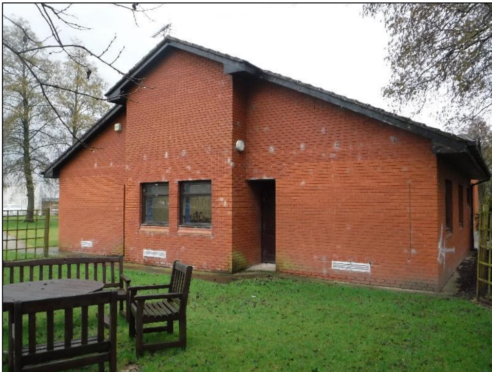
Photo 16 – North gable of Building B15.
