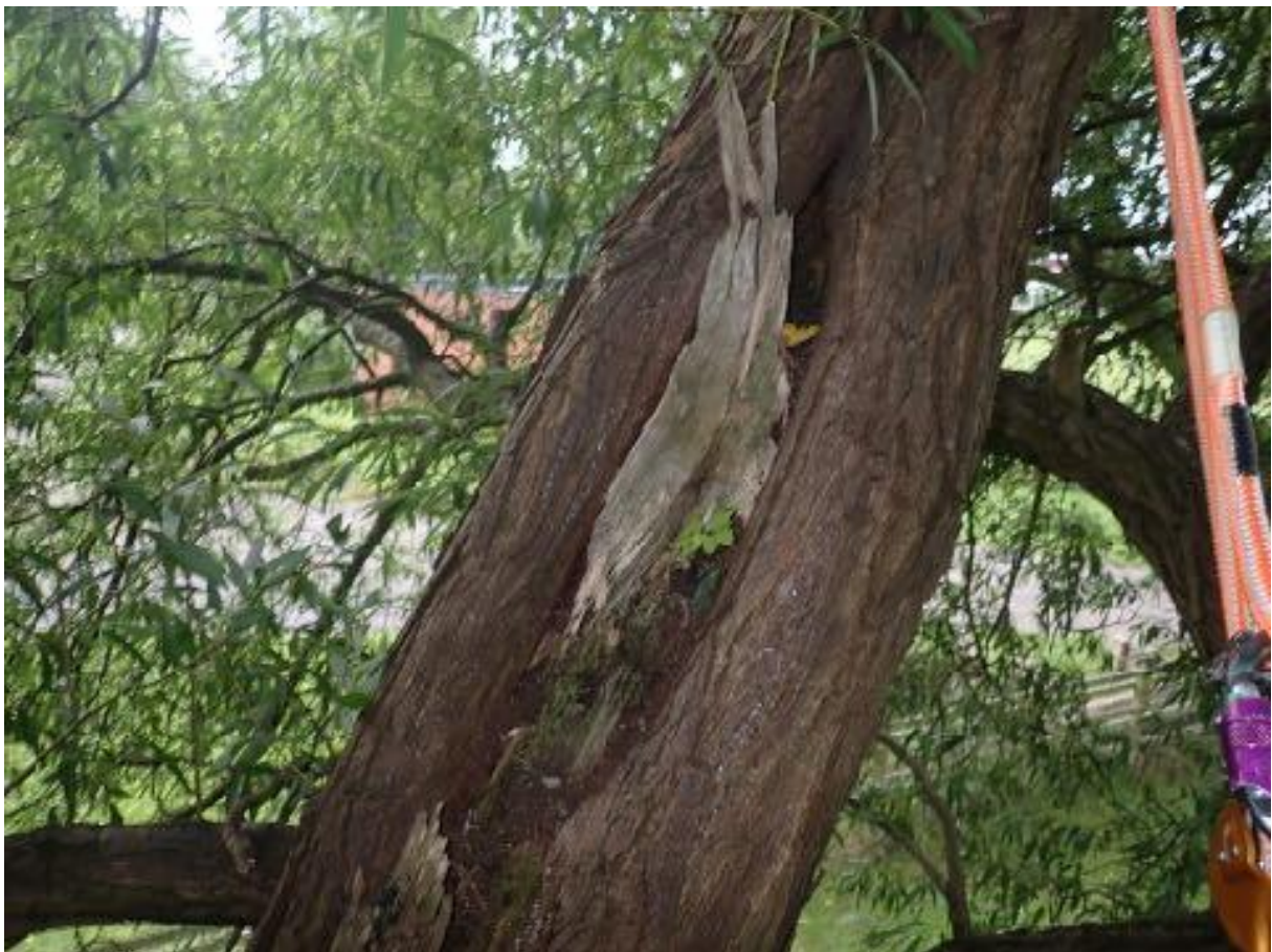
Plate 10 - Tree T2. Tear out on inside of diagonal lead stem at 5m in the west side of the crown. 1m x 20cm of bared heartwood with minor cavity at top of feature with 5cm upward travel. The feature is packed with slugs. No gaps around callus rolls. Negligible.
