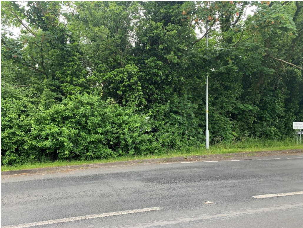
Photograph 4 – Sharp bend sign (left of lamppost) on Ulnes Walton Lane south of Moss Lane obscured by dense vegetation
